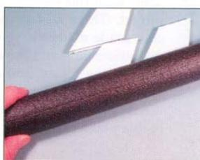
A piece of pipe foam insulation is cut to a length of 14 inches.
