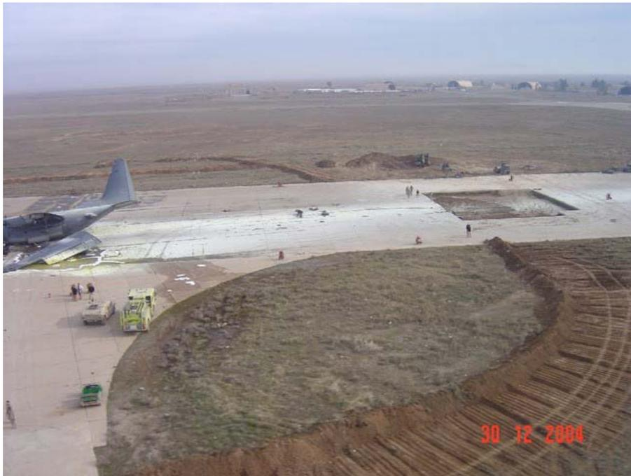
Figure 1: The NOTAM issued for this runway construction project was not accurate, and no signs or lights were in place to warn approaching aircraft. This was an unanticipated threat that created an undesired aircraft end-state (see the C-130 at left).
